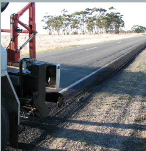
Shoulder repairs in progress
